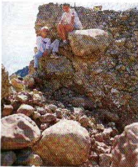
(E) Granular Disintegration is also produced when cementing material in conglomerate and sandstone dissolves so the grains fall apart.
