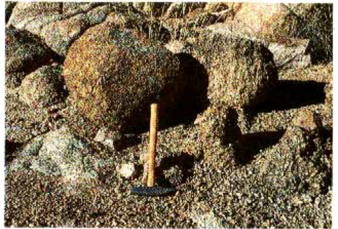
(D) Granular Disintegration is the grain-by-grain breakdown of rock masses. It is common in coarse-grained igneous rocks, sandstones, and conglomerate and results when different minerals in a rock weather at different rates. Feldspars weather rapidly in a granite permitting the quartz grains to slowly separate from one another along their contacts.
